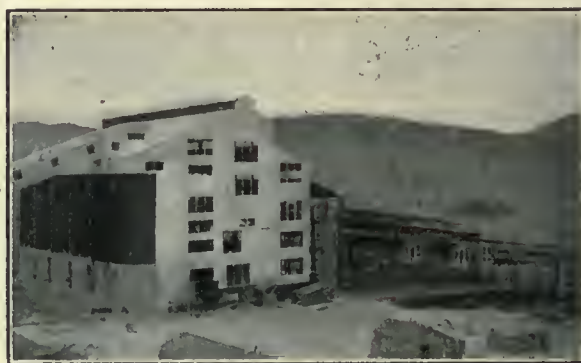
STEEL ORE-BINS ON CONCRETE FOUNDATION, CHINO MILL.
